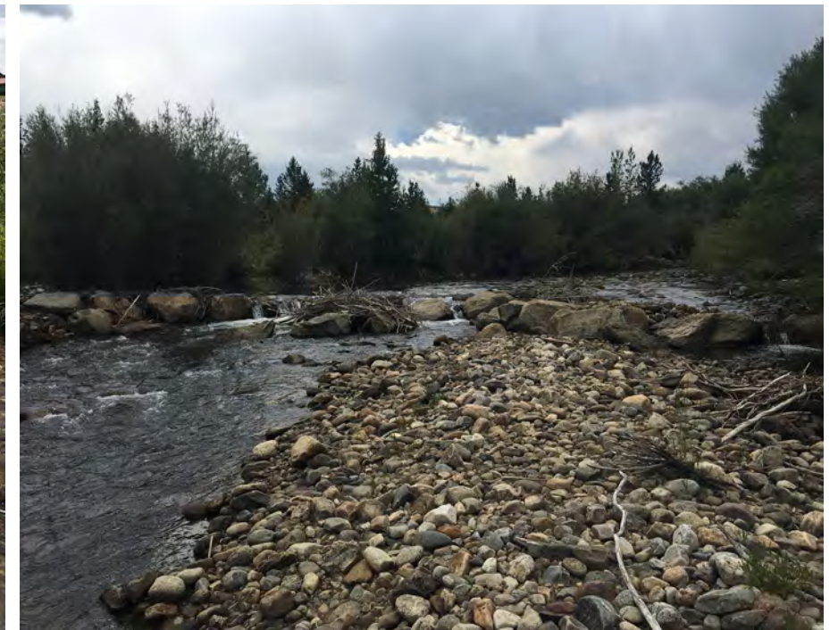
View looking at existing structure requiring maintenance. Regrade cobble bar to allow for pool function.
