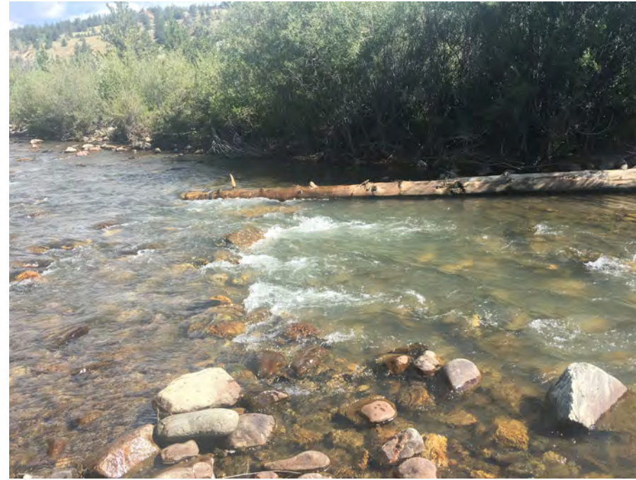
View looking at functional habitat structure upstream of Project Area. Log stabilized with cable and minimal cobble deposition.
