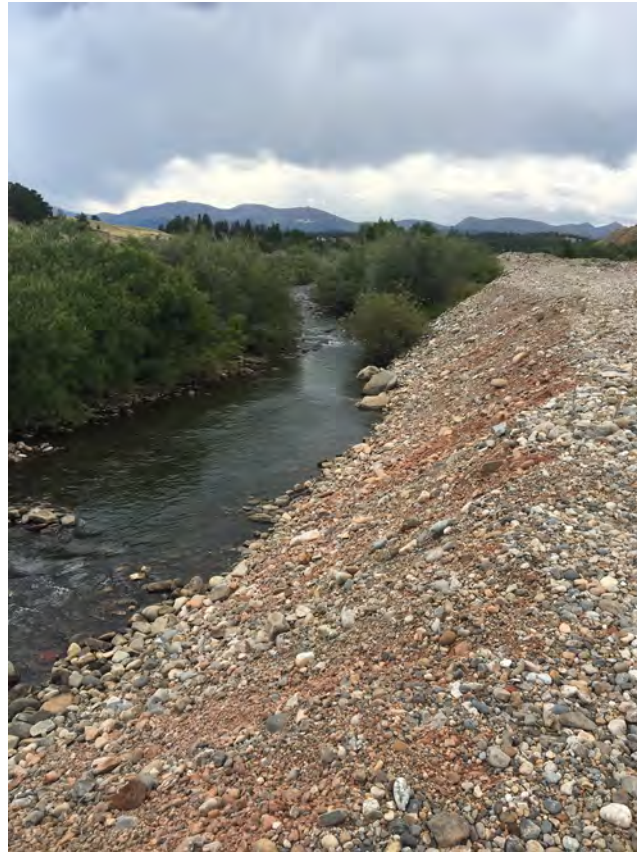
View looking upstream at significantly impaired section of river bank. Highly incised bank is actively eroding. Recommended intervention would be to remove and regrade tailings to stabilize slope. Add riparian plantings to stabilize slope.
