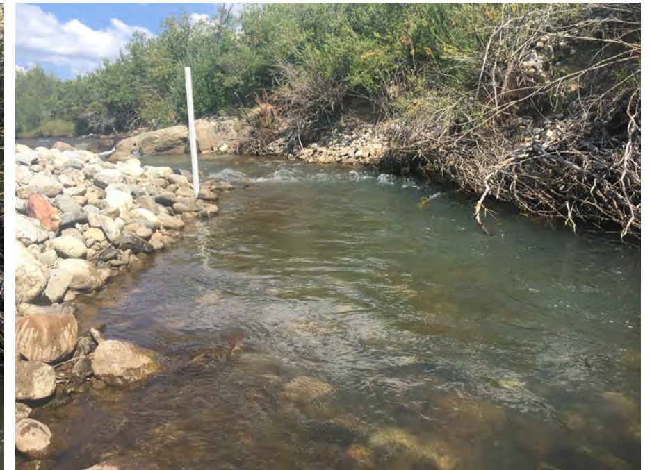
Reduce impacts by regrading cobble deposition and re-align channel.
