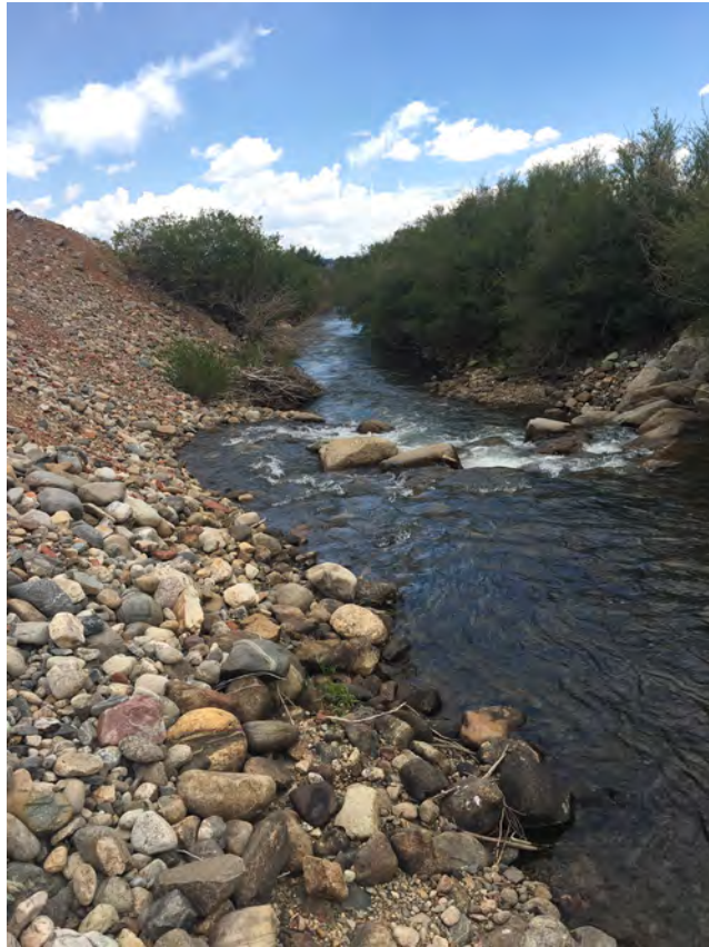
View looking downstream at bank erosion leading to undermining of existing river structure. Recommended intervention would be to remove or regrade tailings to stabilize slope. Key in additional boulders to stabilize structure. Add riparian plantings to stabilize slope.
